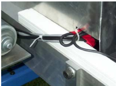
Figure 3.78 Cables entering the front module.
