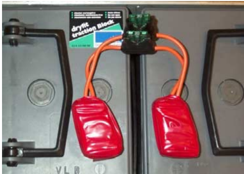
Figure 4.1 For maximum safety the main fuses are placed between the batteries.
