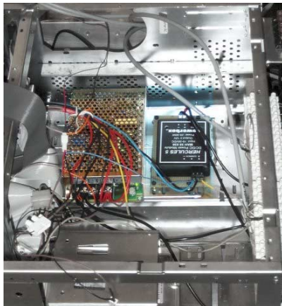
Figure 4.15 The computer supply DC/DC converters mounted in the computer box.
