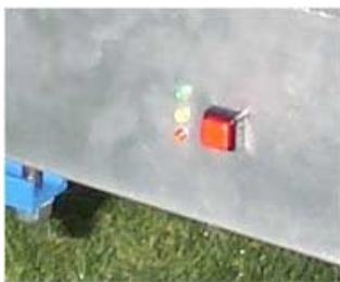
Figure 4.11 Green, yellow and red LED and pushbutton to enable the system.
